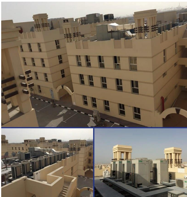
Emirates Flight Staff Accommodation Project Location : UAE Completion : 2014 Outdoor unit : 81 Indoor unit : 521
