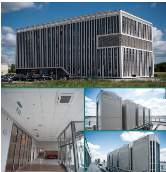
Piotr i Pawel Office Location : Poland Completion : 2016 Outdoor unit : 11 Indoor unit : 92
