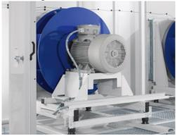
Due to reduced input and output, free-range fans exhibit a high level of operating efficiency. The open construction also guarantees good cleanability and operating safety through the frequency controlled direct drive.
