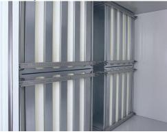
The air's purity is one of the utmost criteria demanded of AHUs in the pharmaceutical industry. A respectively high significance is given to the air filters that have the following duties: The filters protect people from infections as well as the AHUs and the channel network from contamination. Precise filter monitoring prevents the clogging of the filters and permeation of dust. It also reduces the operating costs, as the filters also reduce the pressure drop.
