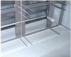
Aerosol test ports effectively support the impact of HEPA filter walls. Beyond that, they enable the monitoring and qualification of HEPA filter walls in a quick and easy manner.
